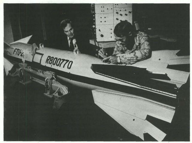
ERB—Chris Dalton and technician Harold Smith (both 1321) work on prototype of extended range bomb being set up for flight test at Tonopah Test Range. ERB incorporates a propulsion unit, canard wings and guidance; it permits stand off delivery of weapon to target.
